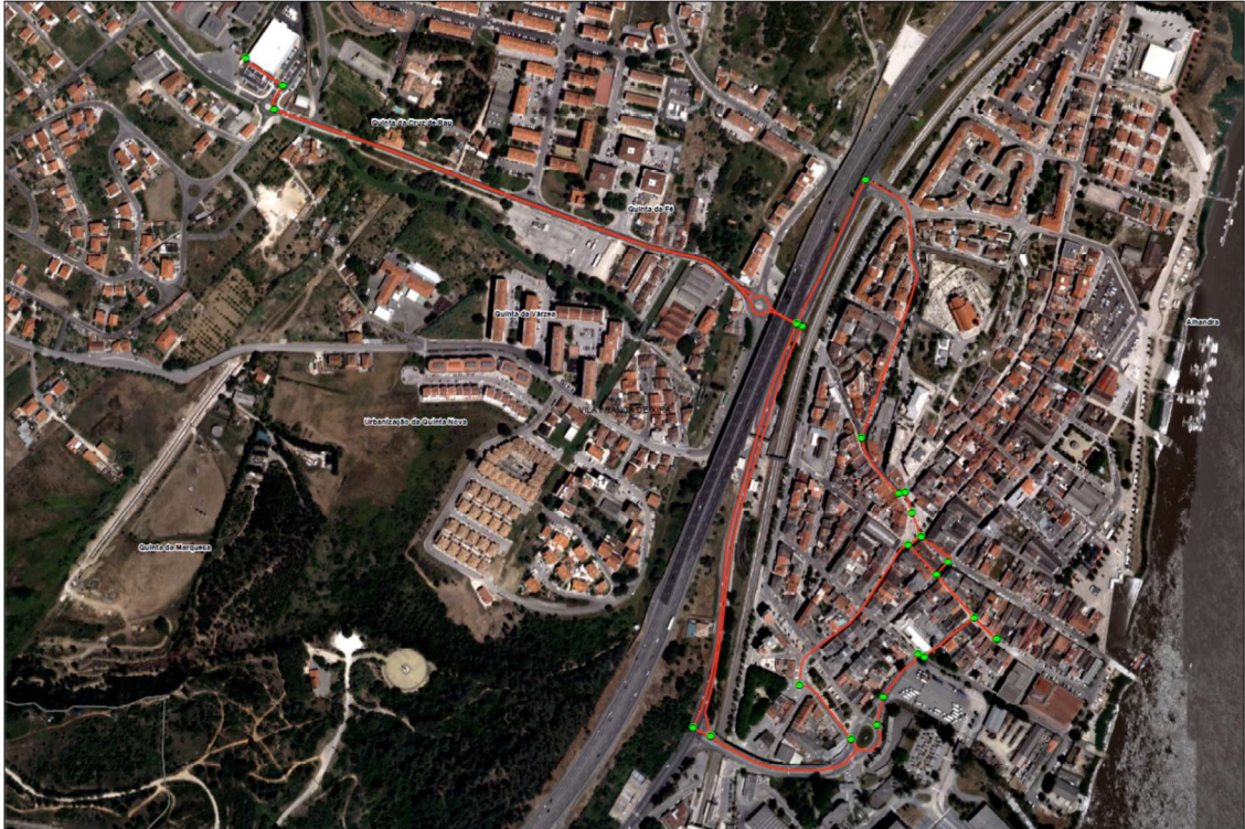
Circuito 1: Alhandra – EB Sobralinho
